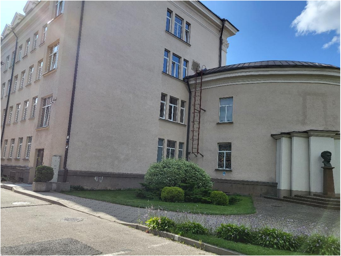
Entrance to the building (Classrooms 209-212)
